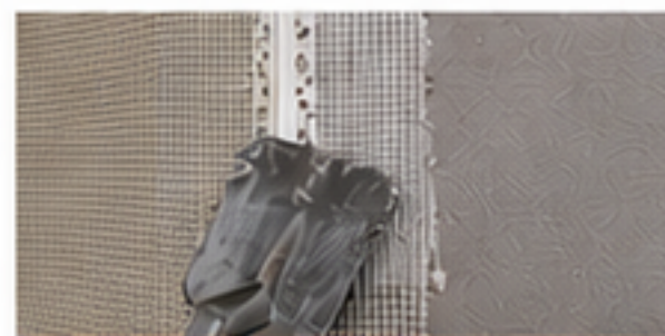
Plaster Reinforcement
